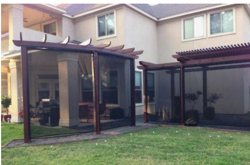
Smaller, individual protection net assemblies incorporated into a trellis structure, and set close to a patio.
